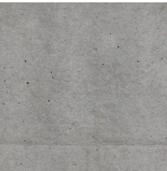
DRIVEWAY SELECTED CONCRETE FINISH - GREY
