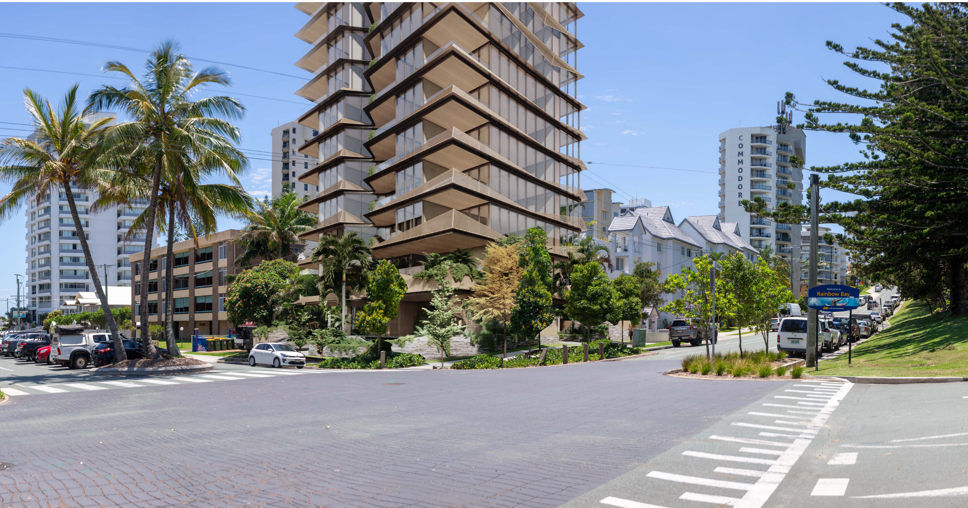
CORNER OF BOUNDARY AND WARD STREET LOOKING EAST
