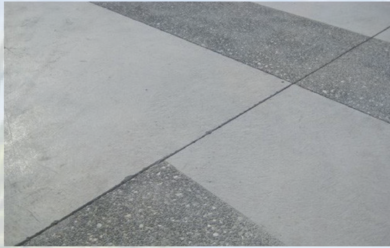
Coloured broom concrete
