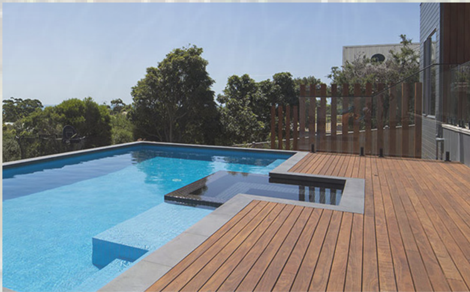
Timber pool deck
