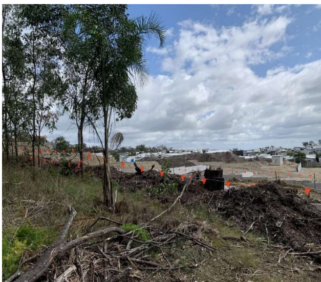
Photo 5: High density residential under construction to the north.
