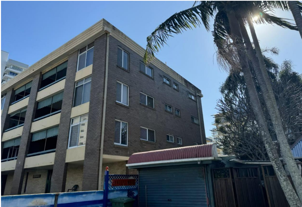
Figure 27: Photo of neighbouring building at 6 Ward Street
