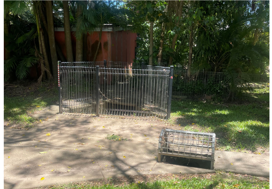
Plate 6 – Stormwater end structure at the rear of the site
