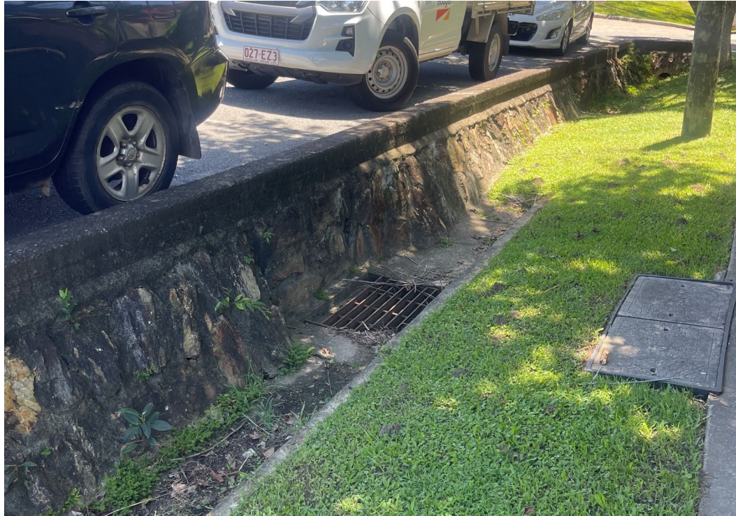
Plate 5 – Drainage gully within the road verge
