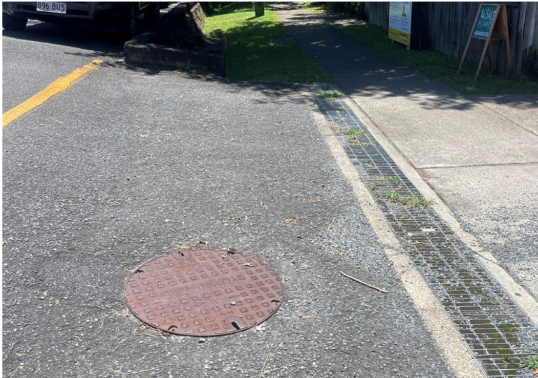
Plate 3 – Sewer manhole within Dutton Street
