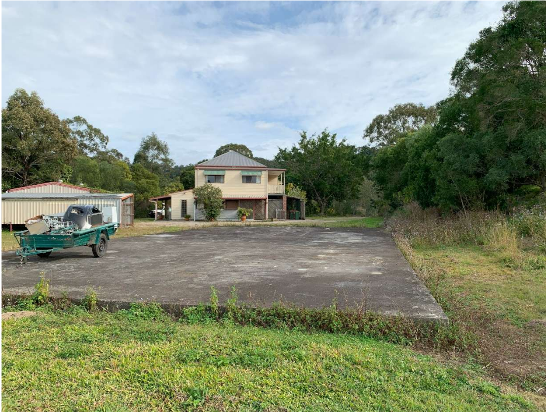
Plate 10 – Cut and fill pad located on hill crest in central portion of the site.
