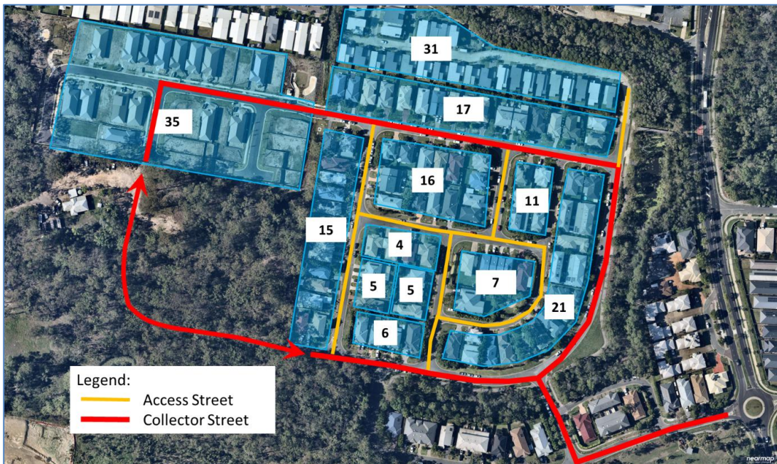
Figure 9.1: Segment of each road in the surrounding road network considered for assessment.
