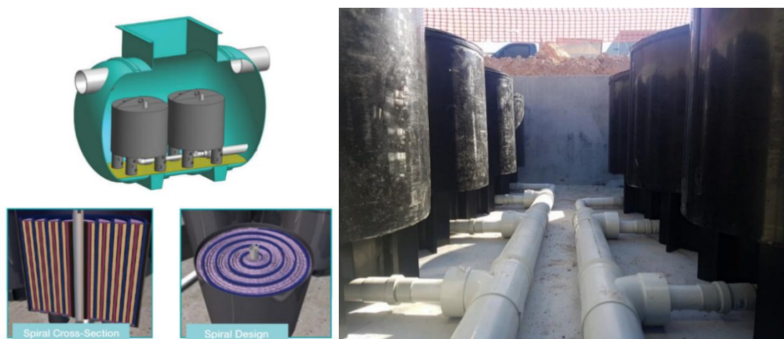
Figure 6.2: AtlanFilter Cartridge Filter
