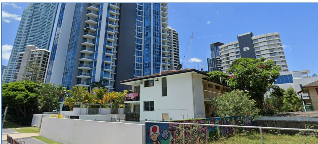
Figure 20: Google street image of the development to the north showing the development turning its back on the proposed development
