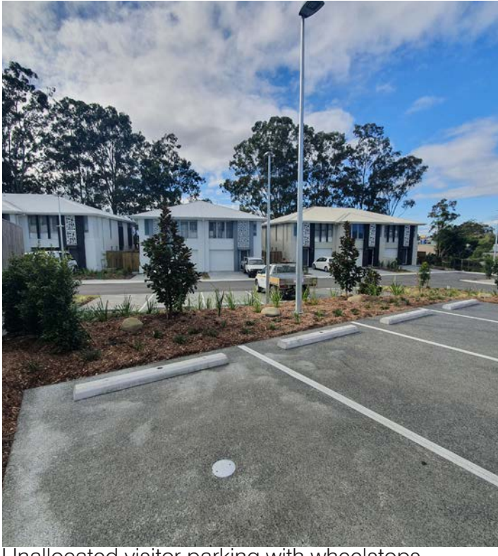
Unallocated visitor parking with wheelstops. Planting adjacent to deter parking on grass.
