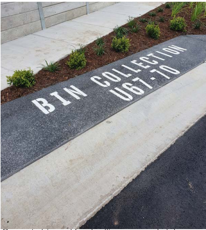
Concrete bin pad for dwellings on road stubs.
