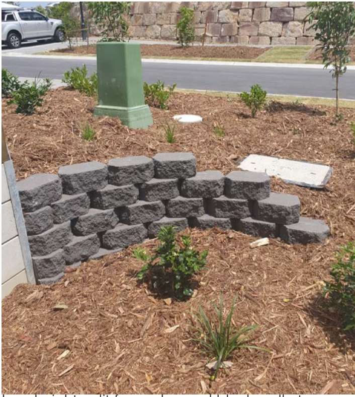
Low height split face, charcoal block wall at frontage to adjust levels between dwellings.
