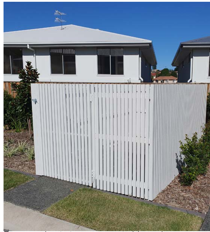
Fence and gate to green waste bin pad, 1500mm high.
