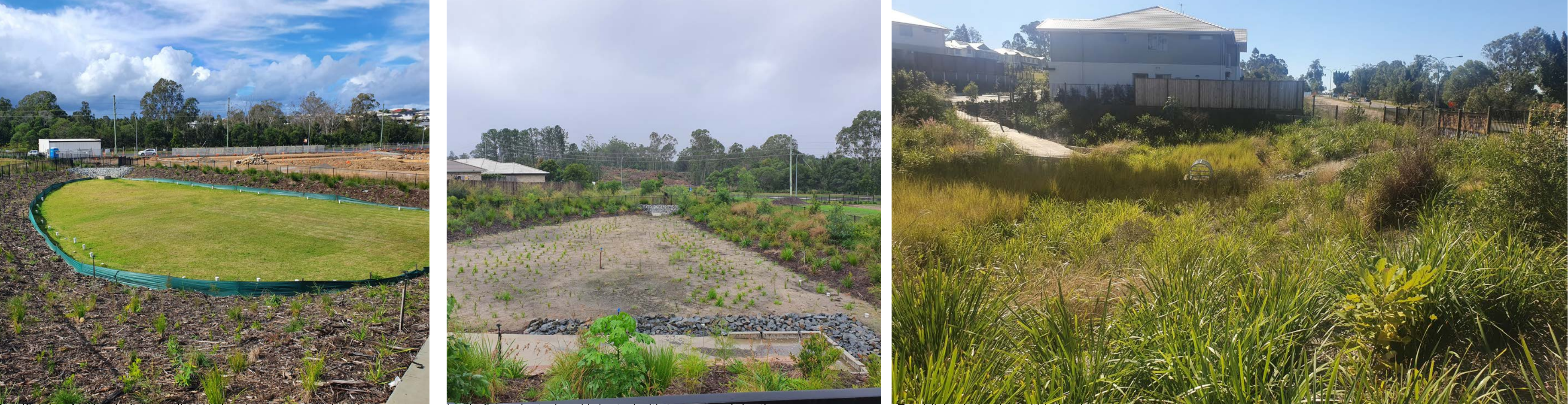
Sacrificial turf to basin floor until 80% development completed. Batters planted earlier. basin floor planted and irrigated with temporary irrigation. Established planting within basin.
