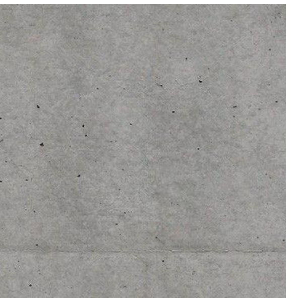
DRIVEWAY SELECTED CONCRETE FINISH - GREY
