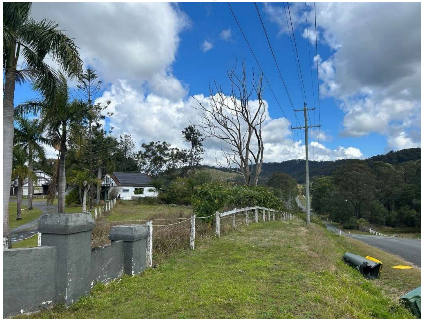
Figure 12 - Courtney Rd frontage - view to south-west
