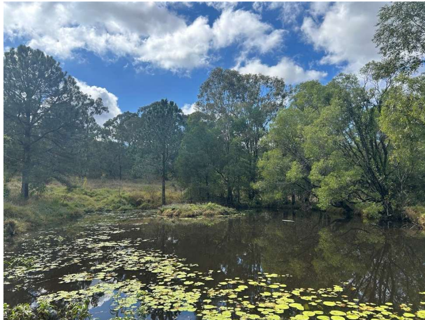
Figure 19 - Constructed dam on subject site
