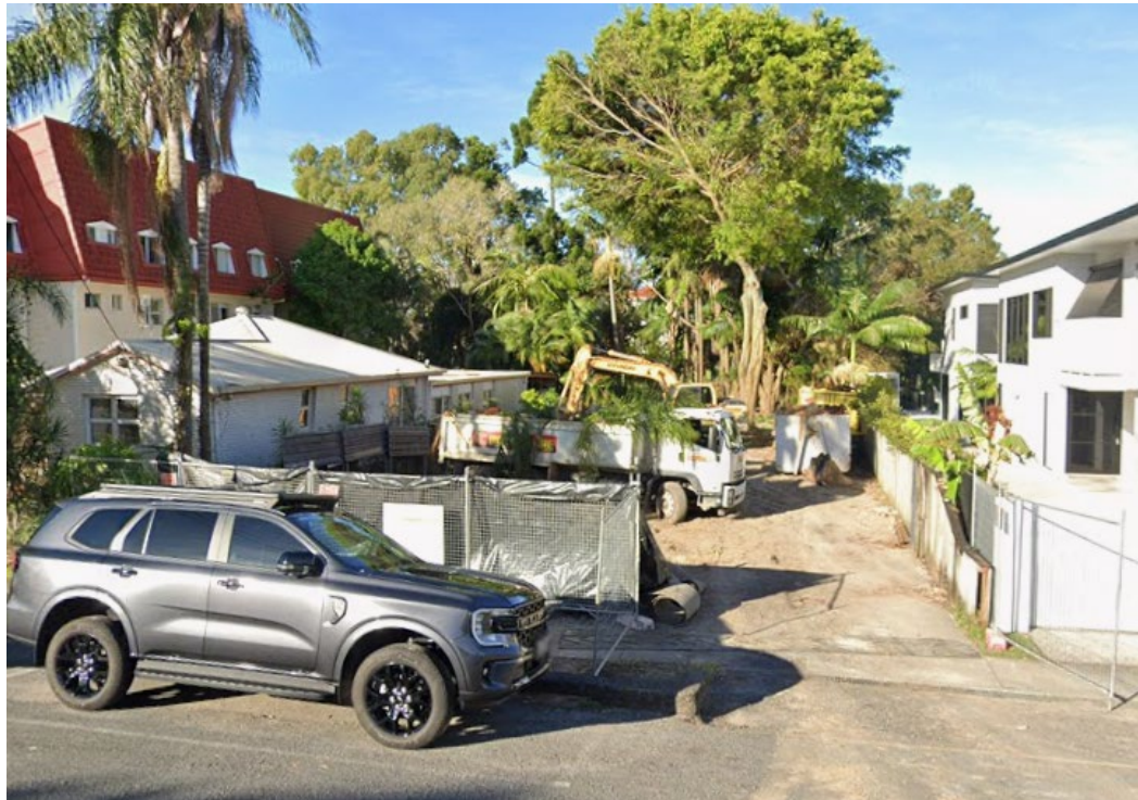
Plate 1 – Site viewed from Dutton Street
