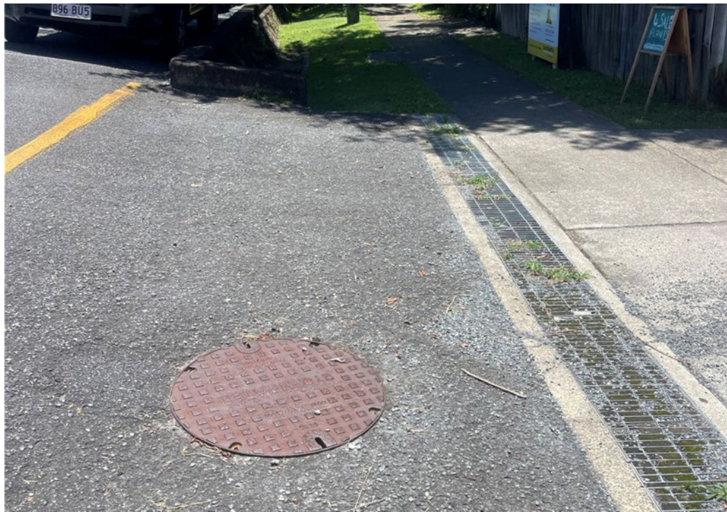
Plate 3 – Sewer manhole within Dutton Street
