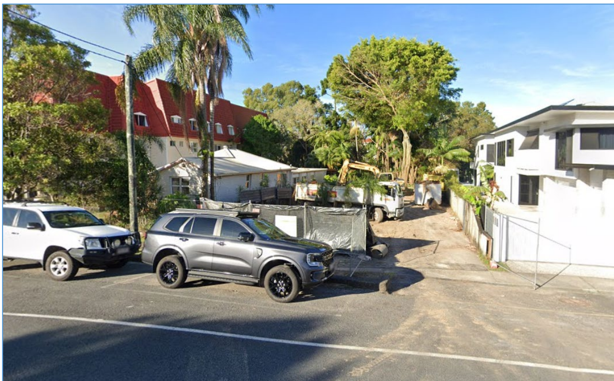
Figure 3.4: Photograph of Site
