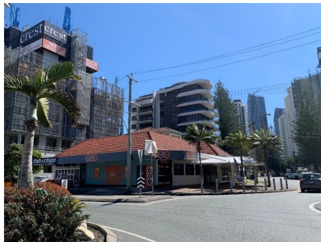
Figure 21: Street view of the subject site from the corner of Old Burleigh Road and Armrick Avenue (CoGC site visit, 4 September 2026)
