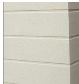
R-3 - RENDERED FINISHED DULUX - VIVID WHITE/ HOG BRISTLE HALF - HORIZONTAL ASHLAR CUTS @300CT
