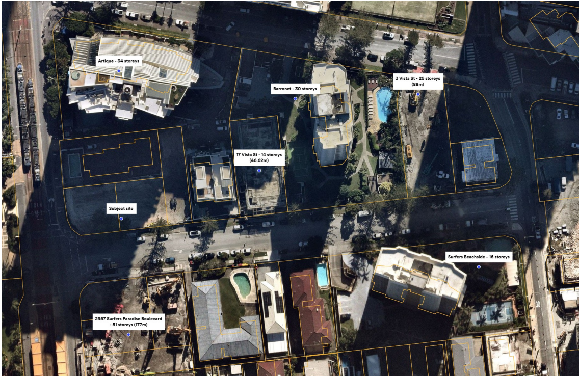
Figure 21. Subject site and surrounding existing and under construction towers (Source: NearMap)
