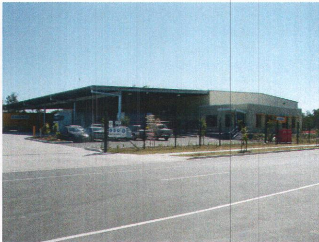
Frame 1 – View of neighbouring Cameron Transport site to the west of subject site.
