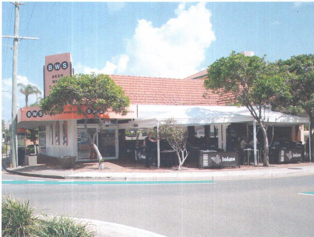
1. Subject site viewed from roundabout on Old Burleigh Road.
