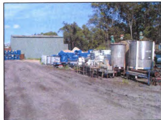
Image 20. Un-bunded storage area
