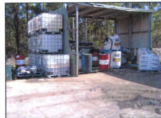
Image 22. Un-bunded storage area
