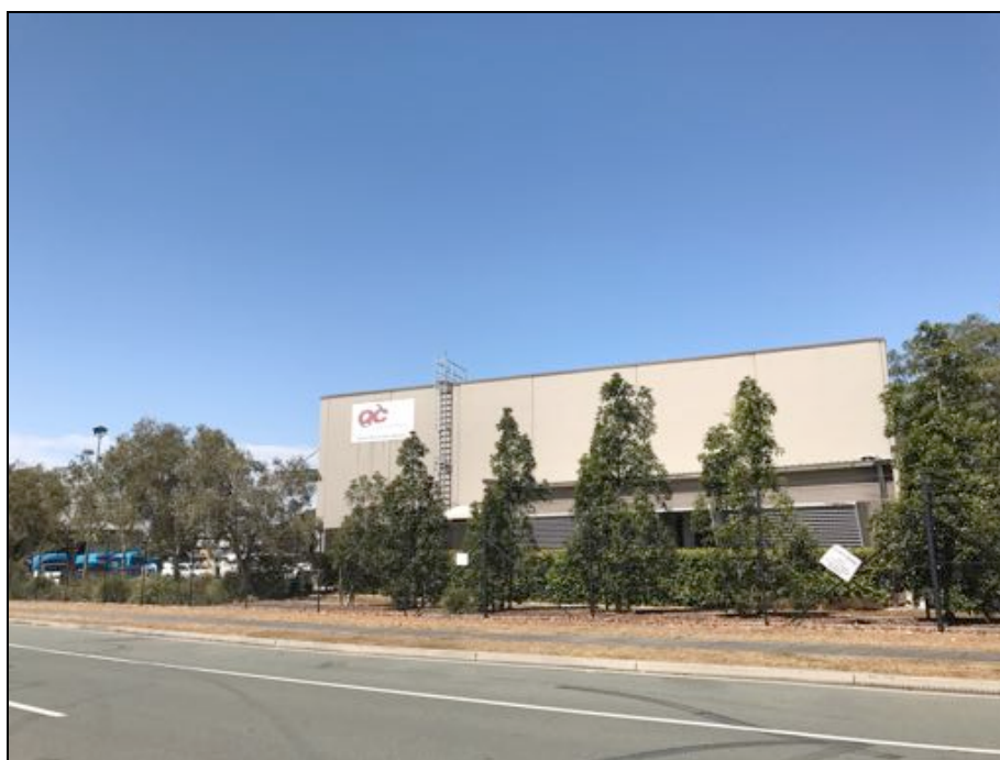
Photograph 13: Existing development on proposed Lot 7 of the reconfiguration which is to have an area of 2,374m 2 . Proposed Lot 7 is currently used by a provider of telecommunications infrastructure. No changes are proposed to the layout or functioning of the development including existing site access or on-site manoeuvring arrangements.
