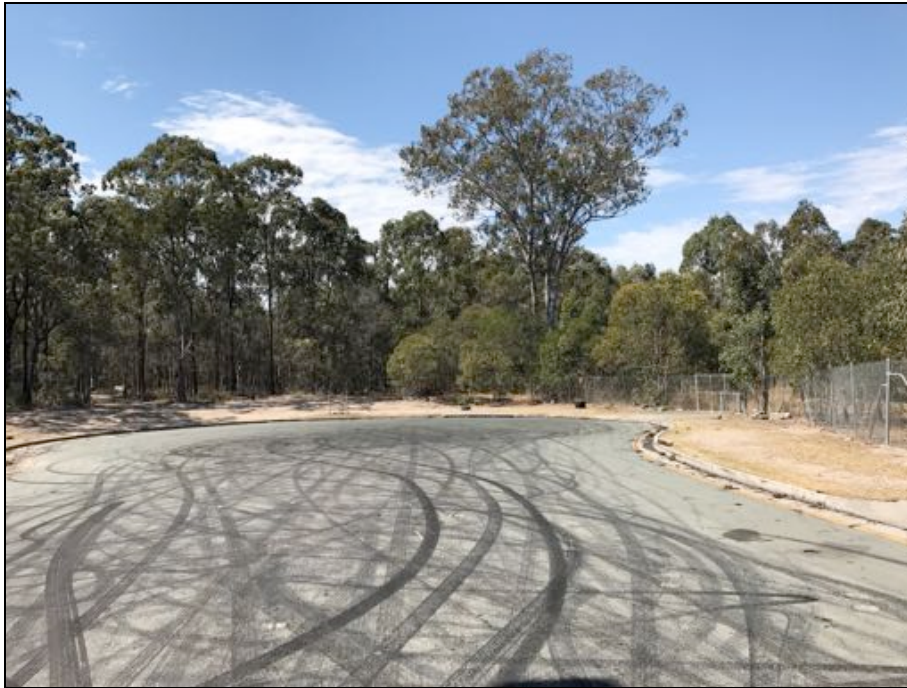
Photograph 4: View east along Christensen Road South to the existing cul-de-sac head at the eastern end of Lot 334 on SP193431. The detention basin for existing industrial developments is located to the southeastern side of Christensen Road South and is to be retained to provide stormwater management for the proposed reconfiguration.
