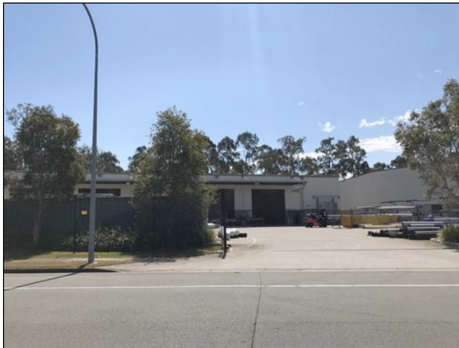
Photograph 12: Existing industrial development on proposed Lot 8 of the reconfiguration which is to have an area of 5,600m 2 . No changes are proposed to the layout or functioning of the developments including existing site access or on-site manoeuvring arrangements.
