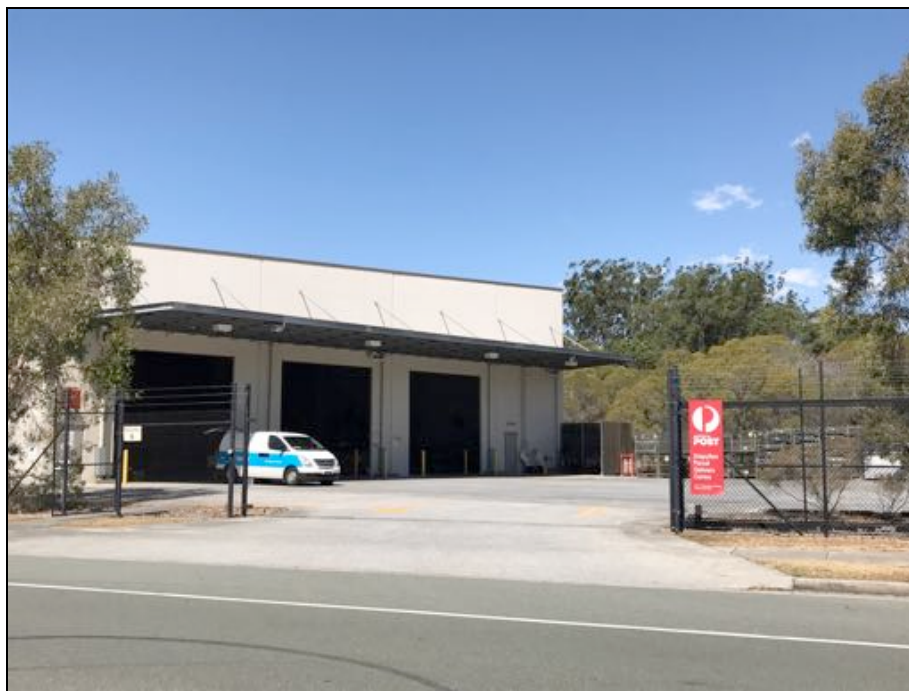
Photograph 14: Existing development on proposed Lot 6 (3,461m 2 ) of the reconfiguration. Proposed Lot 6 is currently used as an Australia Post parcel depot. No changes are proposed to the layout or functioning of the development including existing site access or on-site manoeuvring arrangements.
