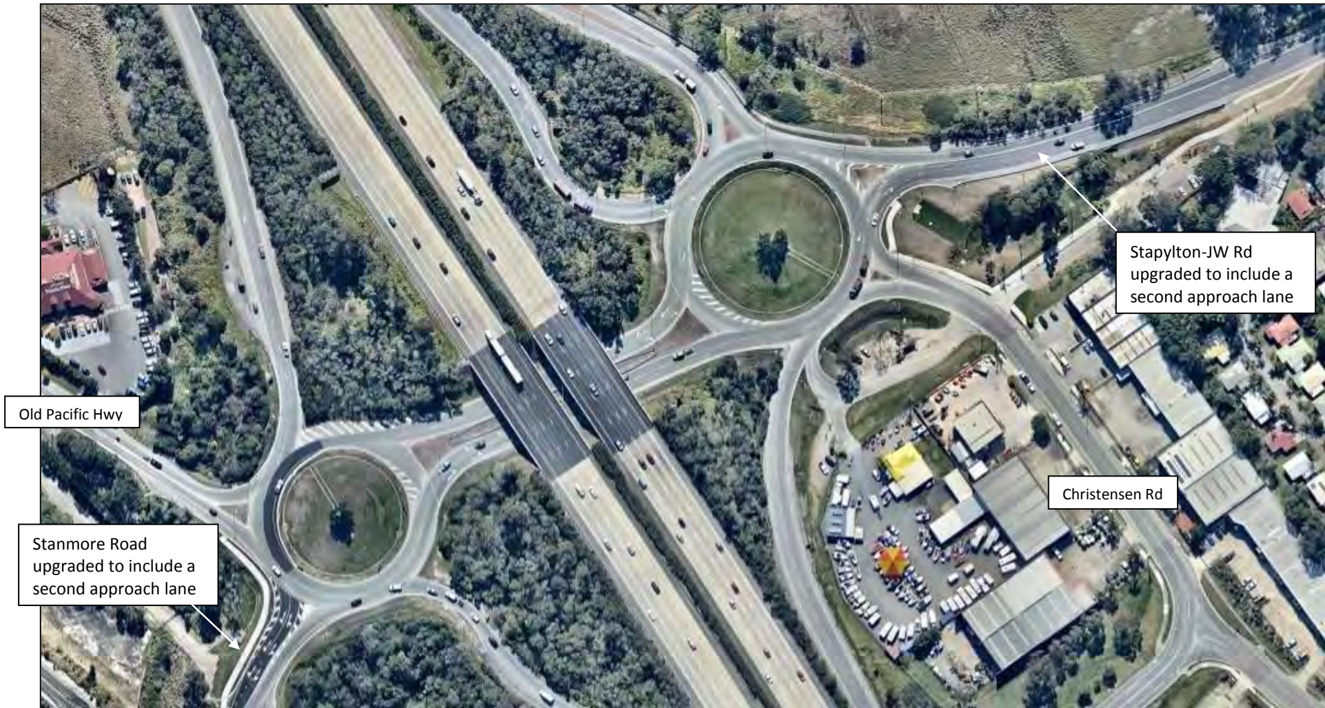
FIGURE 3.1 – EXISTING YATALA NORTH INTERCHANGE (PHOTO AUGUST 2015)
