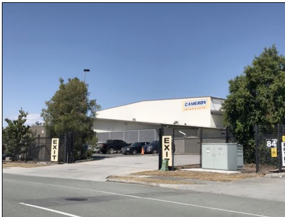
Photograph 5: Existing industrial development located opposite the subject site in Christensen Road South.
