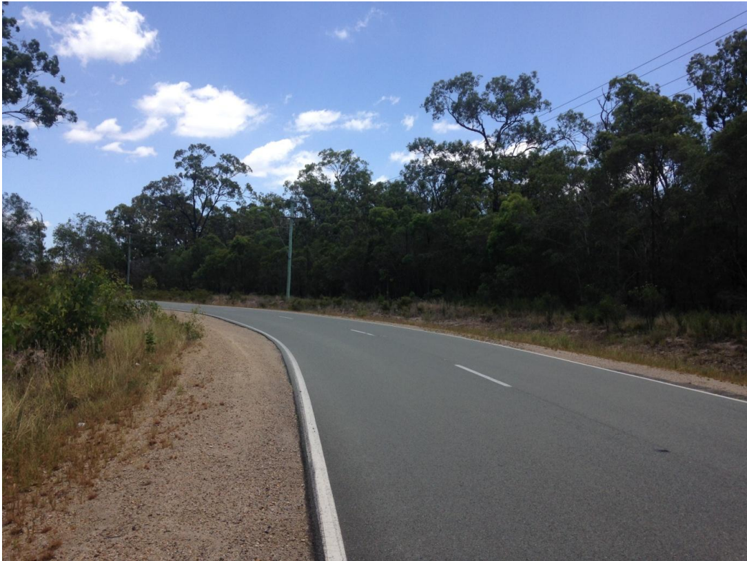
Photo 11 – View of Christensen Road South looking north west toward subject site.
