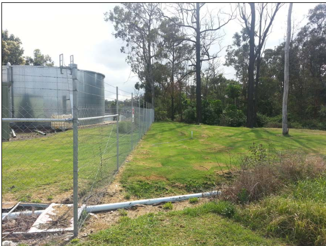
Photo 2 – View looking north-east along the southern boundary of existing Lease A
