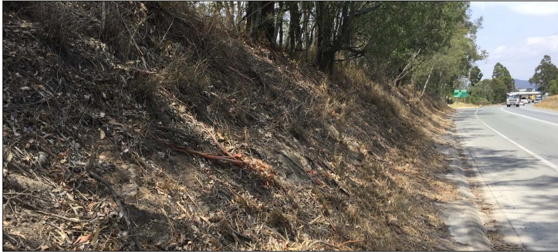
Figure 10 Cut batter looking southwest
