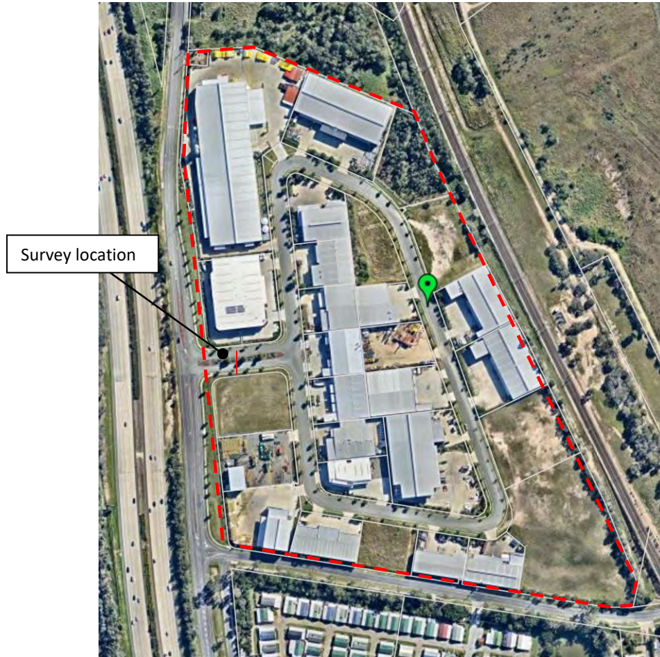
Surveyed site at Motorway Circuit, Ormeau
