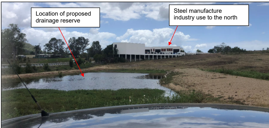
Figure 6: Photo looking towards the north of the site (Source: Site photo taken 10 December 2020)
