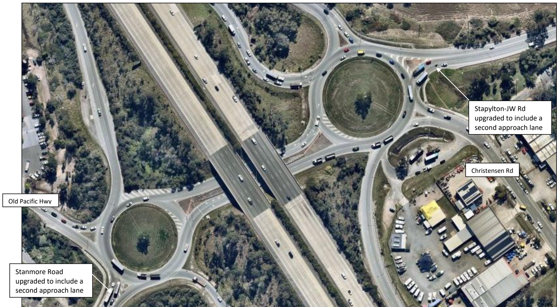
FIGURE 3.1 – EXISTING YATALA NORTH INTERCHANGE (PHOTO AUGUST 2020)
