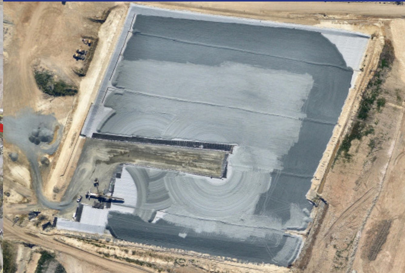
Stapylton Landfill Facility
