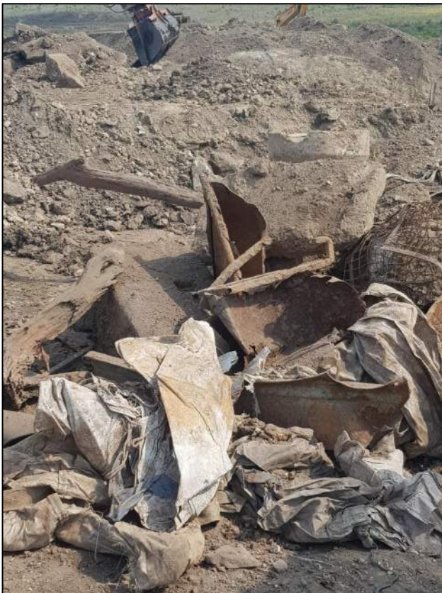
Figure 6: Debris removal during rehabilitation works (December, 2019)
