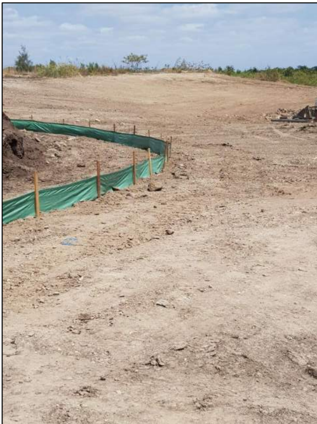
Figure 12: General earthworks (December, 2019)
