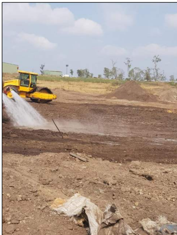
Figure 10: General earthworks (December, 2019)
