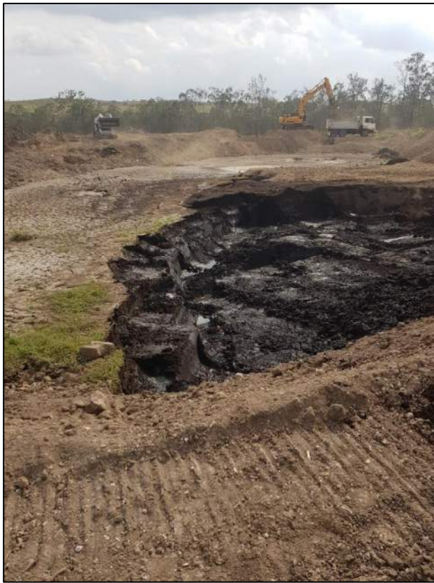
Figure 9: Removal of unsuitable subgrade (December, 2019)
