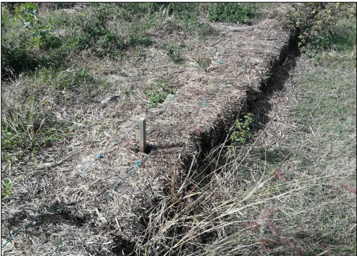
Figure 18: Hay Bale Sediment Control and Filtration (August, 2020)
