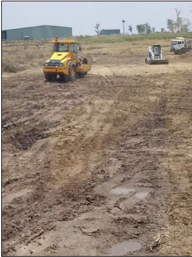
Figure 11: General earthworks (December, 2019)
