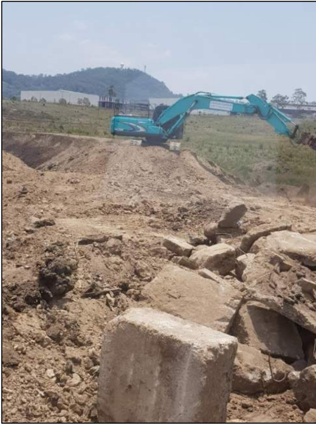
Figure 7: Concrete block removal during rehabilitation works (December, 2019)
