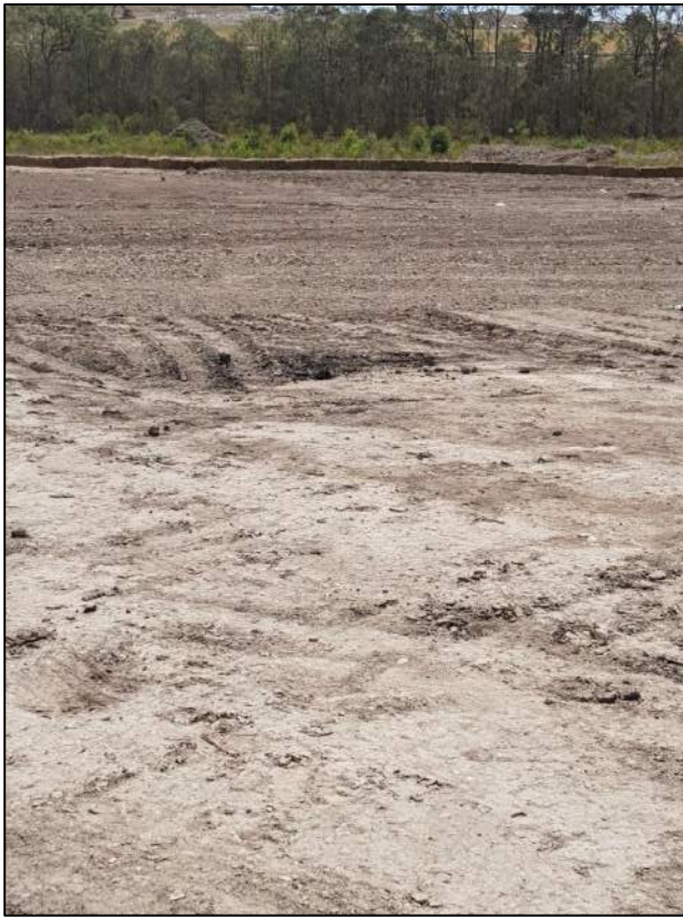
Figure 13: General earthworks showing hay bales as sediment and erosion control (December, 2019)
