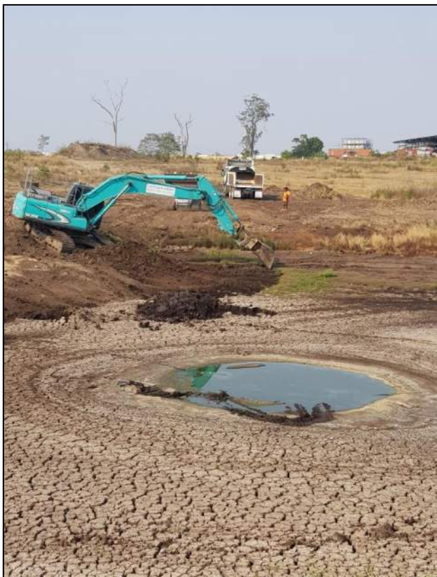
Figure 8: Removal of unsuitable subgrade (December, 2019)
