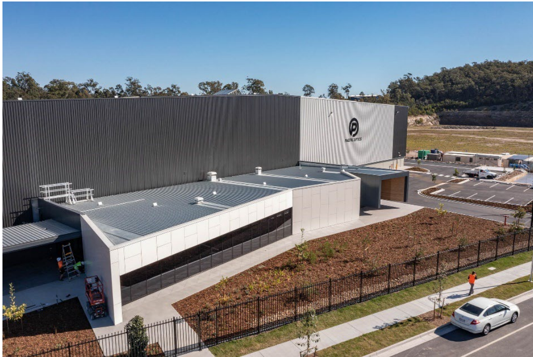
Figure 22 – Example of FPI Queensland Architectural finish (GDP file, 2022)
