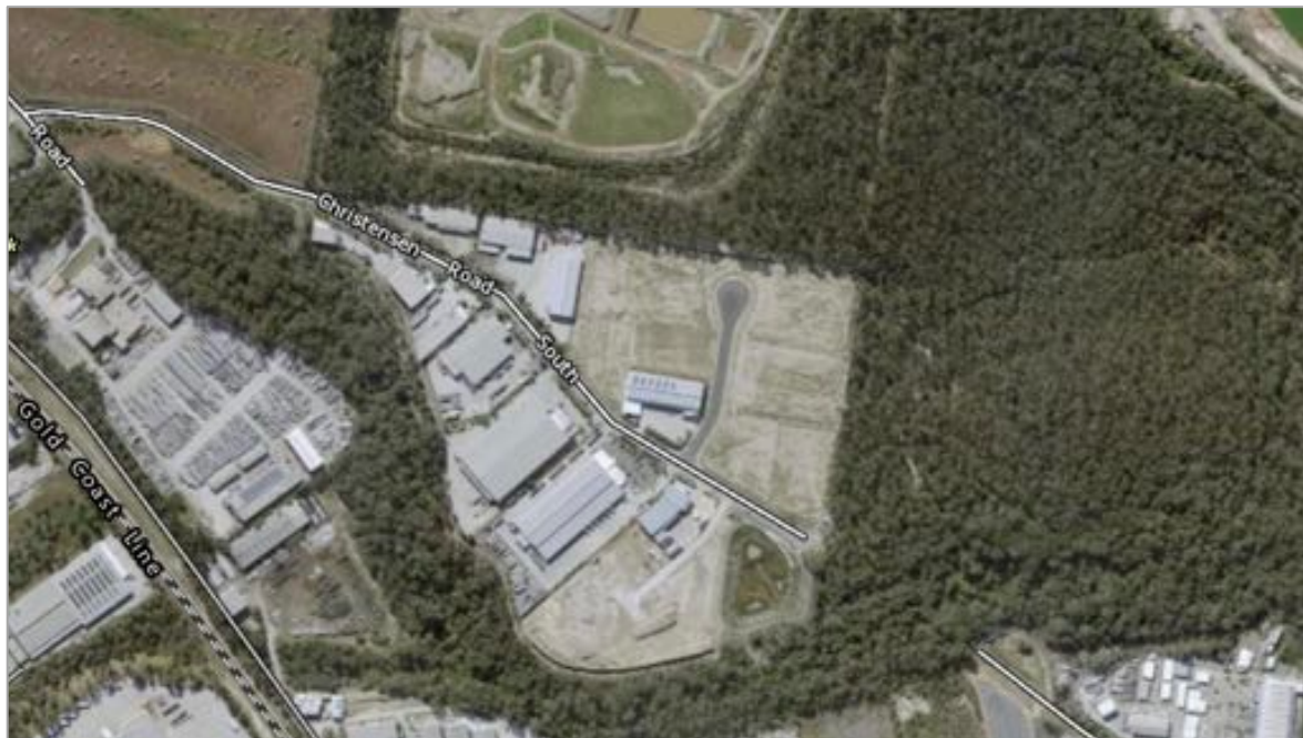
Photograph 1: Aerial image of subject site and newly constructed road (Proximity Place) within the approved industrial estate. Whilst the survey plan is currently before Council for plan sealing, all civil works associated with the original subdivision approval including bulk earthworks, new road, services and stormwater detention / treatment have been completed.
