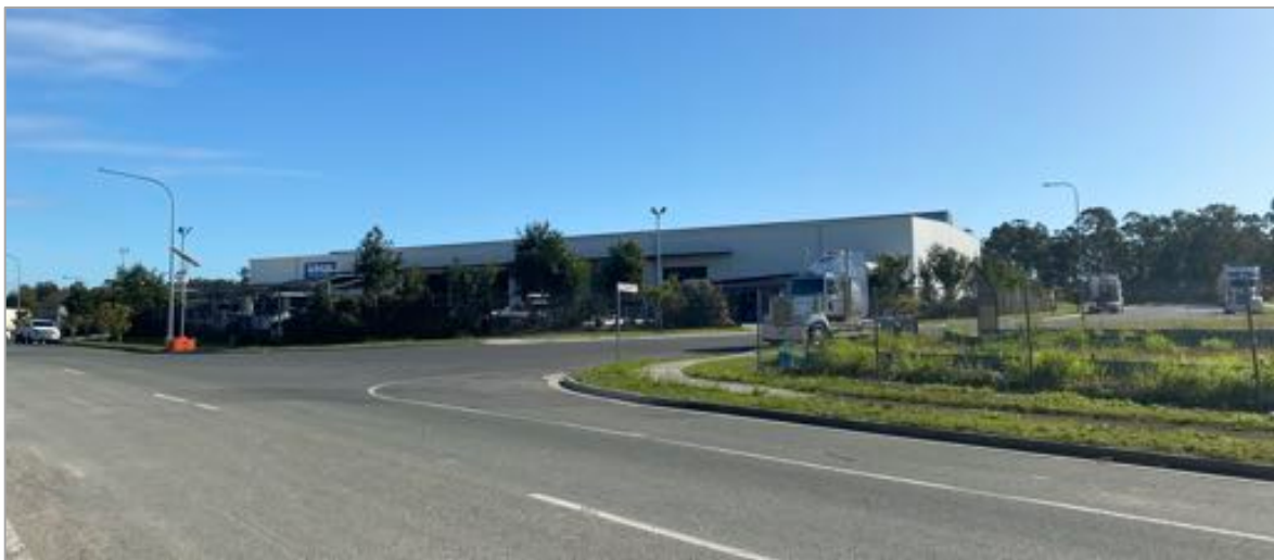
Photograph 4: View of newly constructed intersection at Christensen Road South and Proximity Place.
