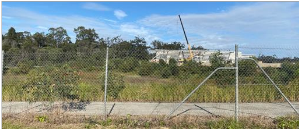
Photograph 5: View of newly constructed wetland area to the south of Christensen Road incorporating stormwater bioretention works which is sized to treat all stormwater runoff from both the new road and industrial lots.
