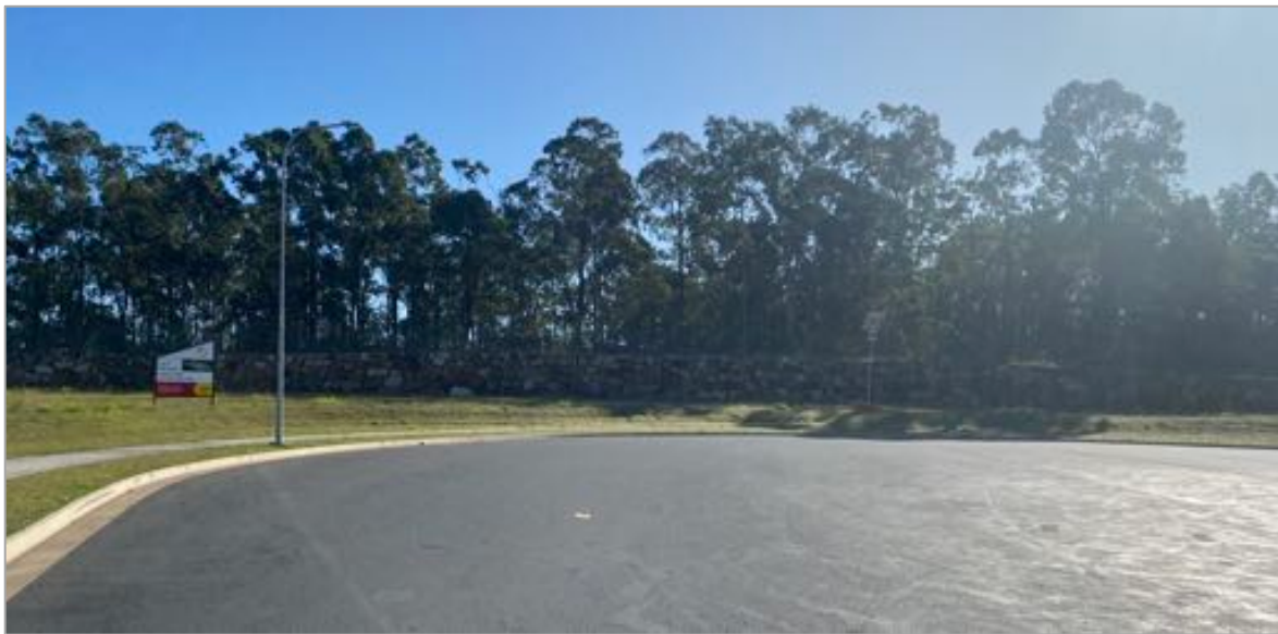
Photograph 3: View of finished industrial lots to the north and retaining walls along the boundary which adjoins the Stapylton Landfill facility.
