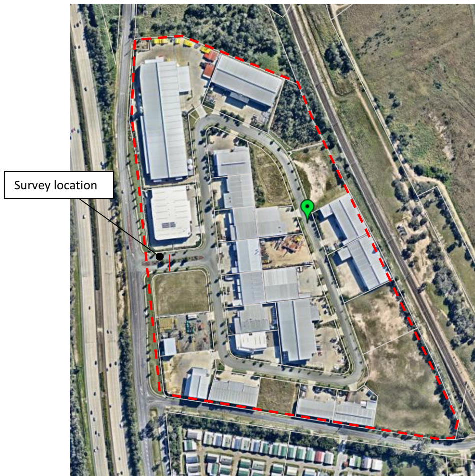
Surveyed site at Motorway Circuit, Ormeau
