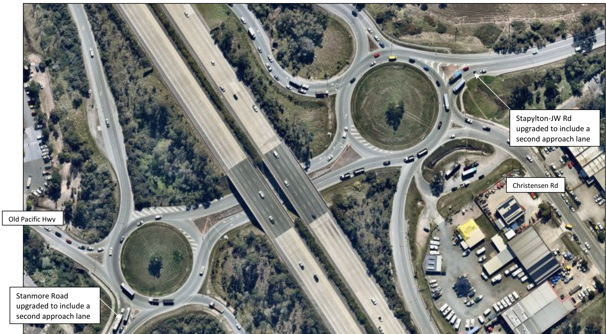
FIGURE 3.1 – EXISTING YATALA NORTH INTERCHANGE (PHOTO AUGUST 2020)
