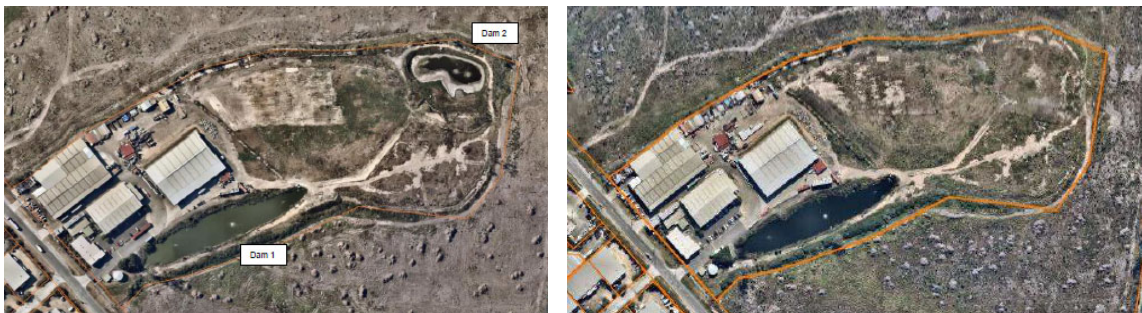
Figure 3: Lot 500 before rehabilitation works (left) and after rehabilitation works (right) (Source: Icubed Consulting)
