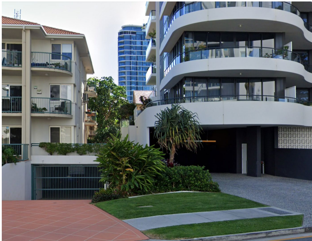
Figure 13 – Subject site (left) and northern adjoining development interface (right). Source: Google.
