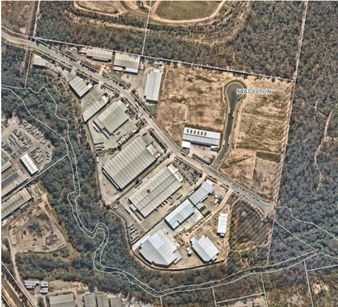
Figure 5: Aerial of subject site (pre plan sealing)
