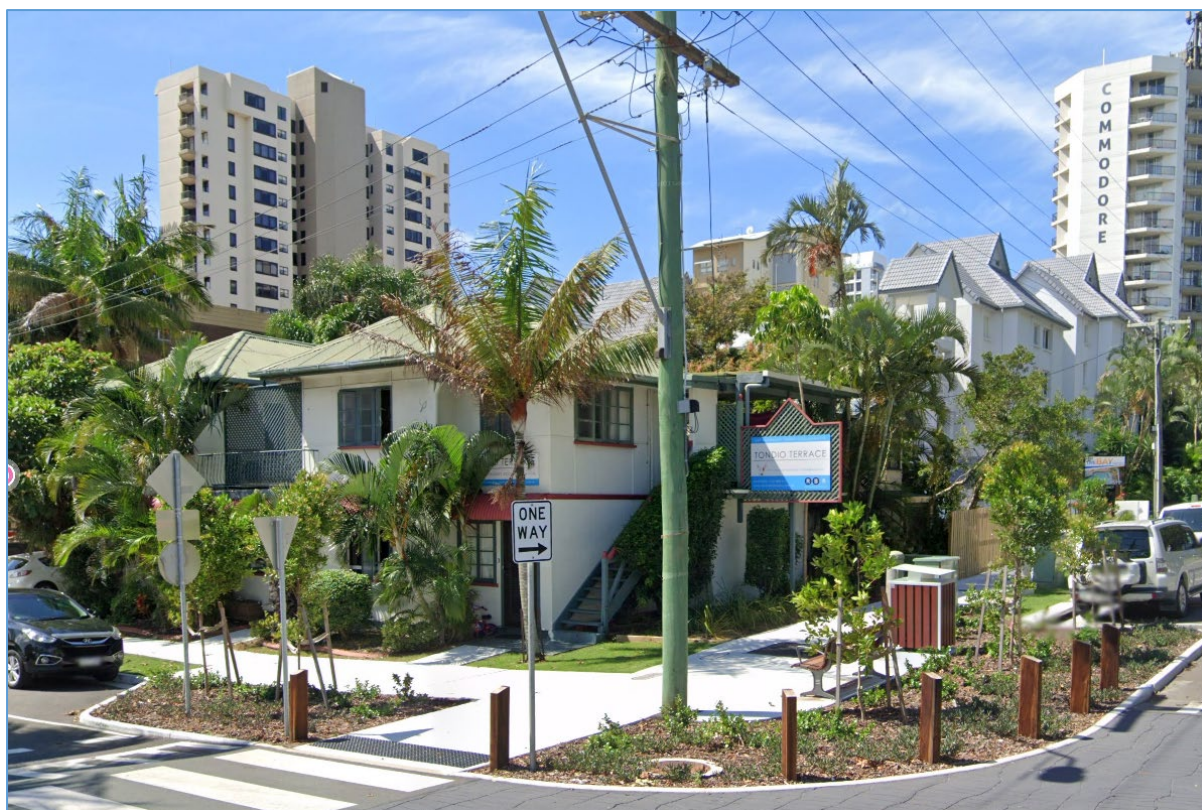
Figure 3.5: Photograph of Site
