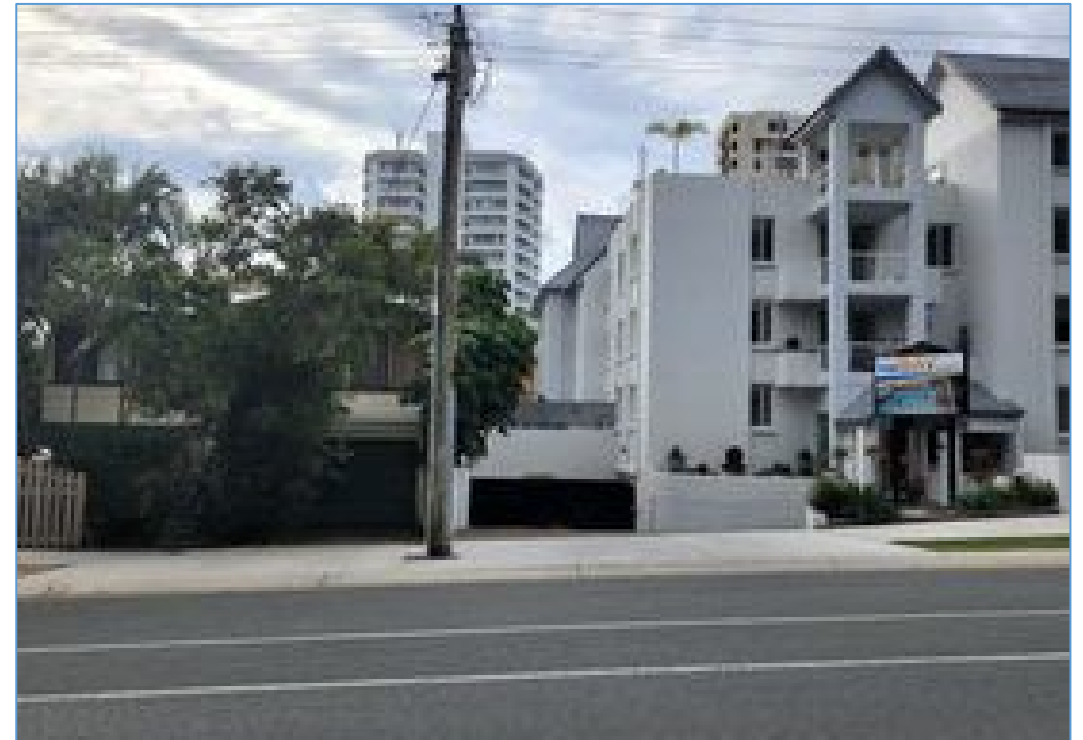
Plate 8 – Boundary interface to east (Boundary Street)
