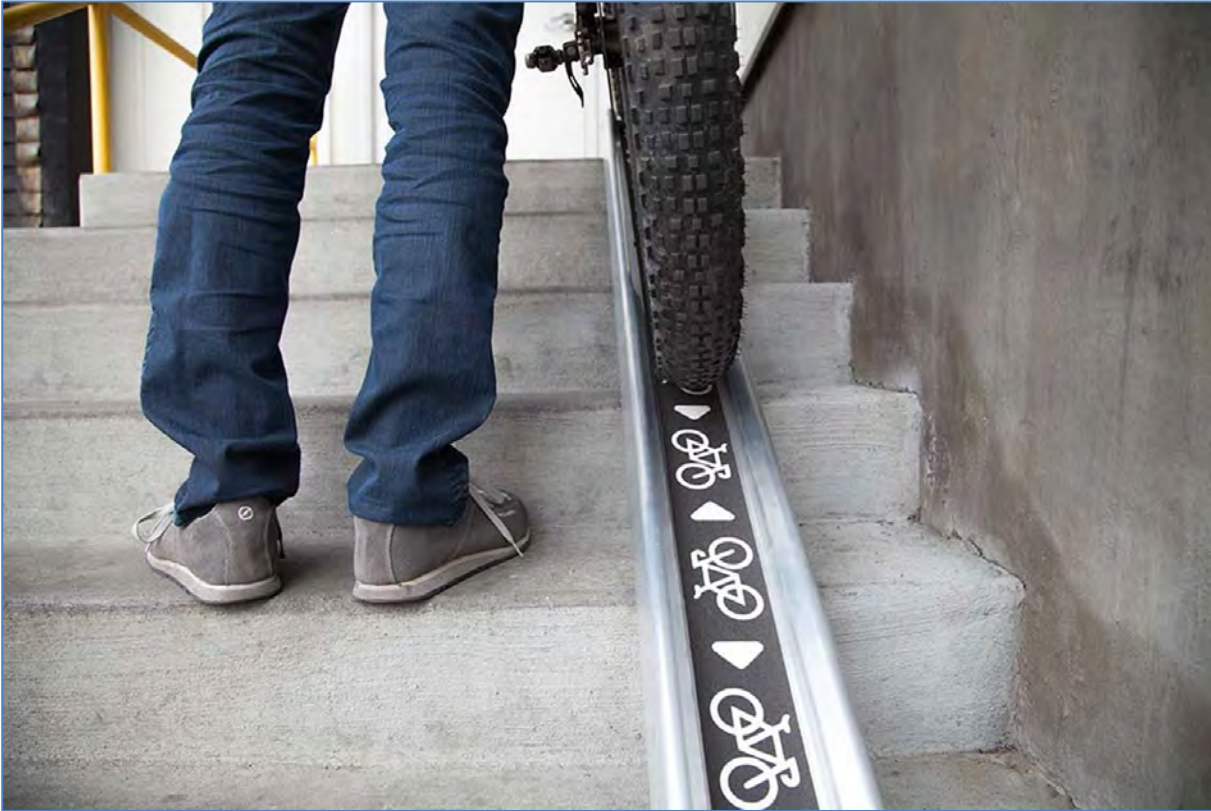
Figure 7-1: Example of stairway bike groove
