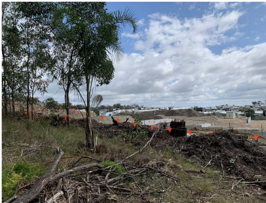
Photo 5: High density residential under construction to the north.
