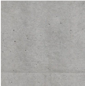
DRIVEWAY SELECTED CONCRETE FINISH - GREY
