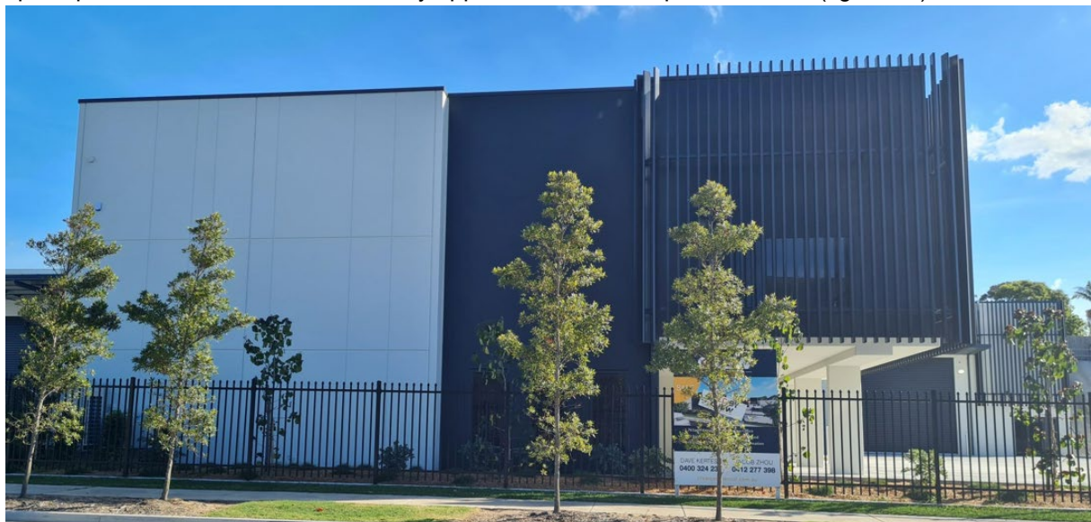
Figure 10: Existing industrial building and established frontage landscaping (Source: City officer)
