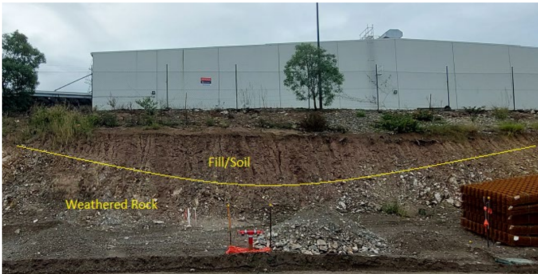
Image 1: Northern batter area requiring treatment
