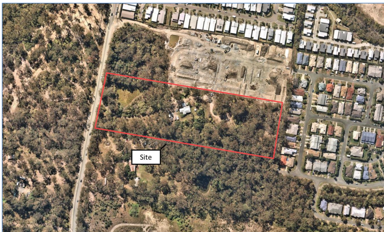
Figure 1.2: Site aerial view
