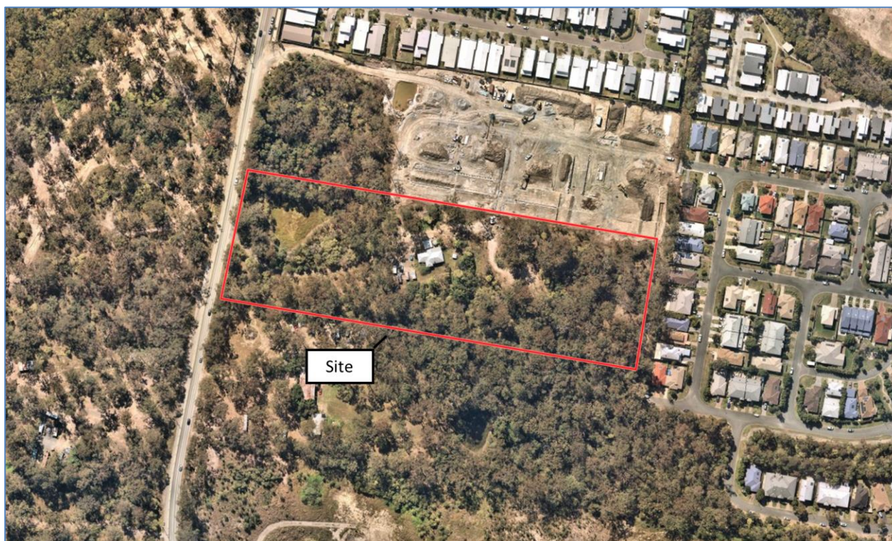
Figure 1.2: Site aerial view
