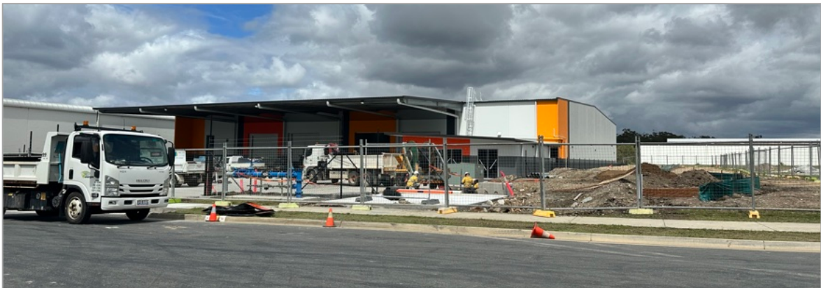
Photograph 3: View of approved High Impact Industry use currently under construction and directly opposite the subject site.
