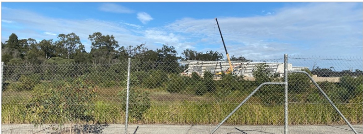
Photograph 5: View of newly constructed wetland area to the south of Christensen Road incorporating stormwater bioretention works which is sized to treat all stormwater runoff from both the new road and industrial lots.
