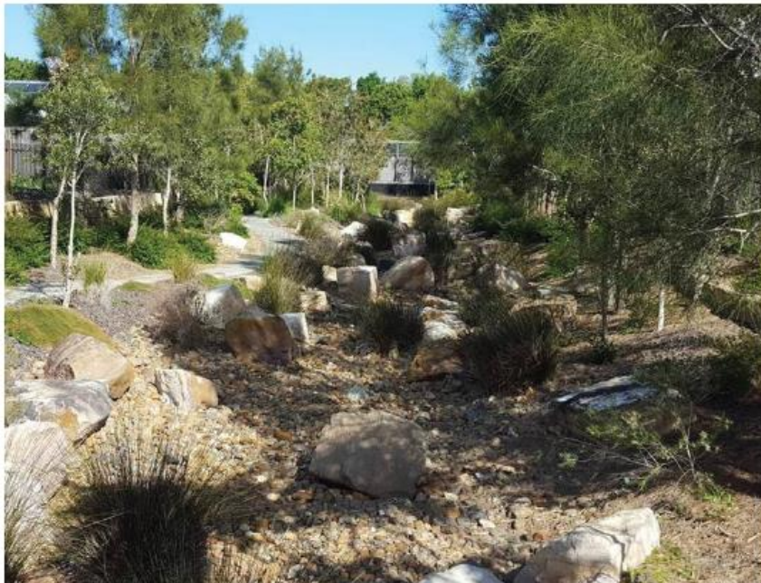
Example Image of Rock Lined Swale
