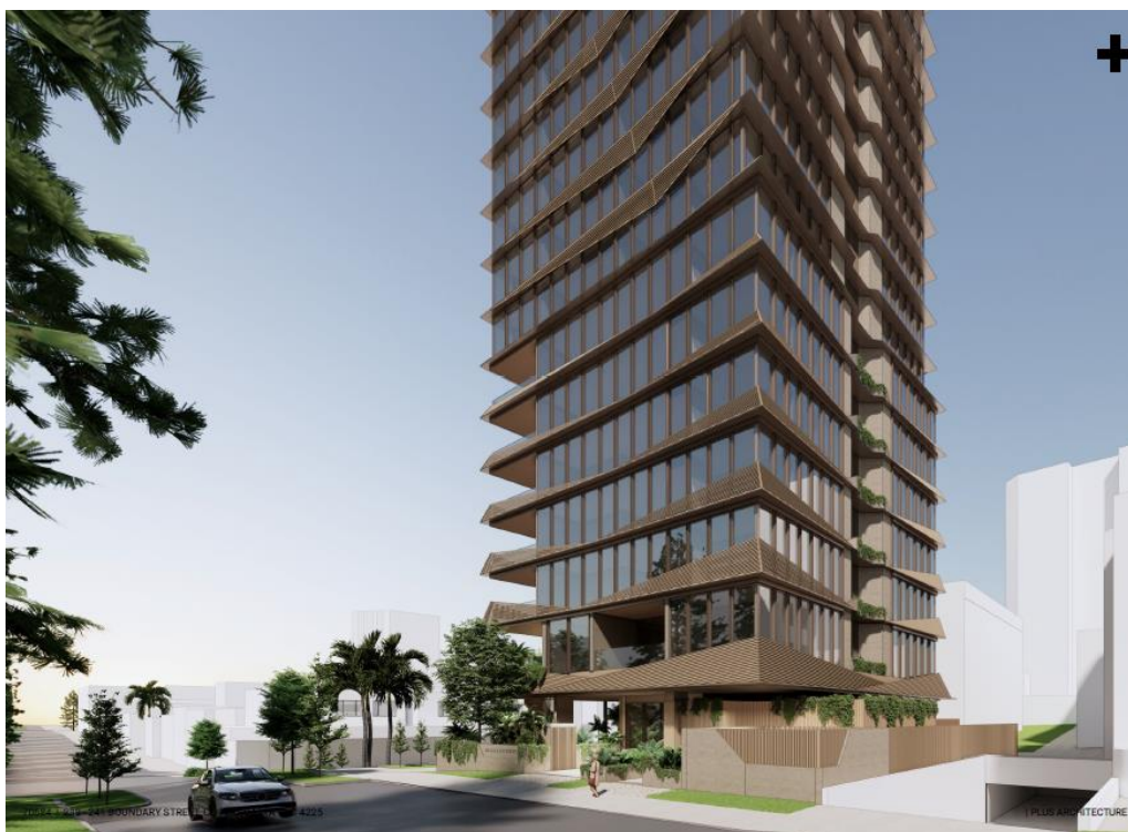
Figure 7: Feature screens to the upper levels (Plus Architecture)
