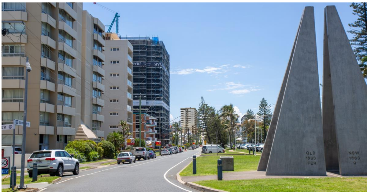
Figure 5: Corner of Boundary and Clarke Street looking east (Plus Architecture)
